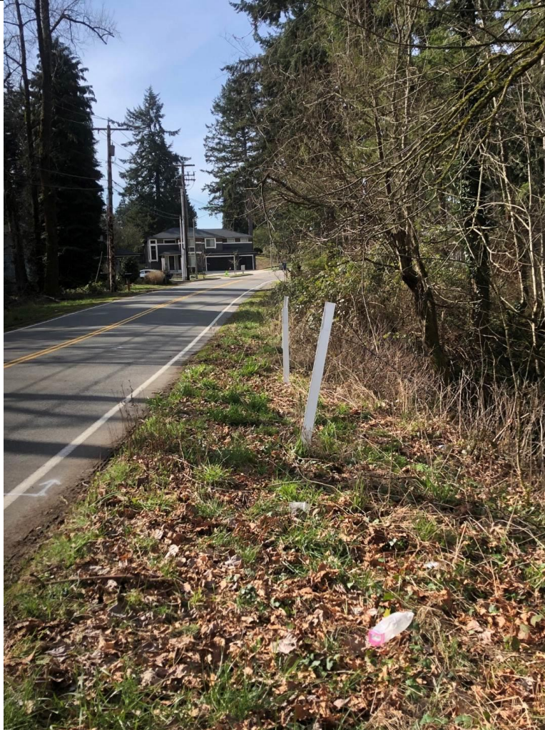
Plate 1 – Facing west along the north shoulder of SE May Creek Park Drive from the east side of the Gypsy Creek ravine.
